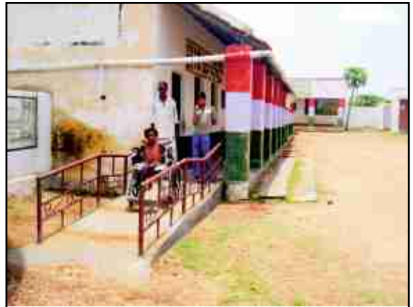
School Accessibility - Ramps and Railings to facilitate easier access
